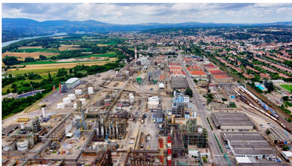
Figure 103. The Roches-Roussillon chemical platform.
