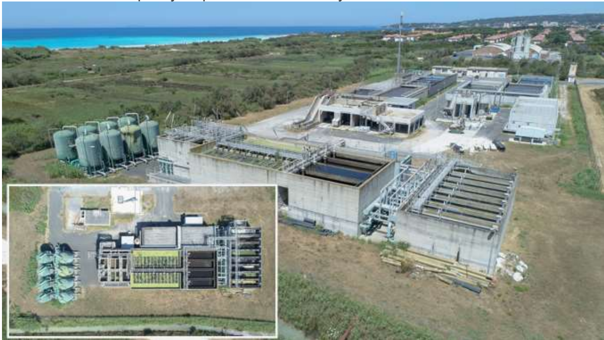
Figure 30. ARETUSA WRP in Rosignano WWTP Area.
