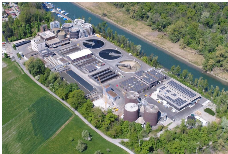
Figure 12 Aerial view of WWTP Altenrhein
