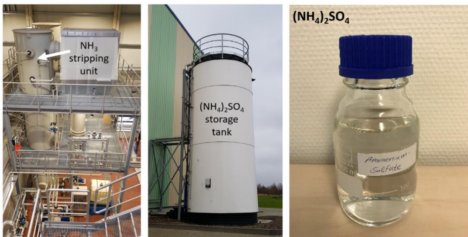
Figure 42 Pictures of the ammonium sulphate production units, the storage tank and an ammonium sulphate solution sample
