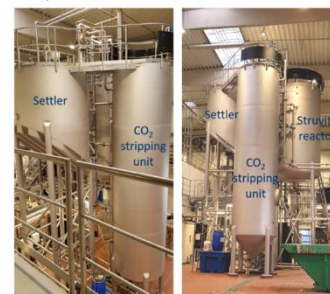
Figure 95 Phosphorus recovery technologies in NextGen with feed concentrations or contents
