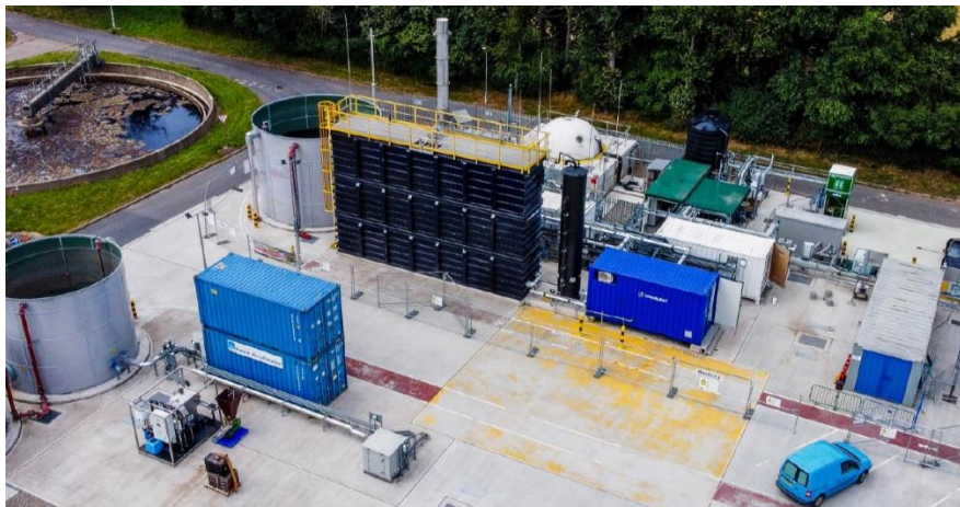
Figure 7. Aerial picture showing the NextGen demonstrator including the anaerobic membrane reactor and degassing unit.
