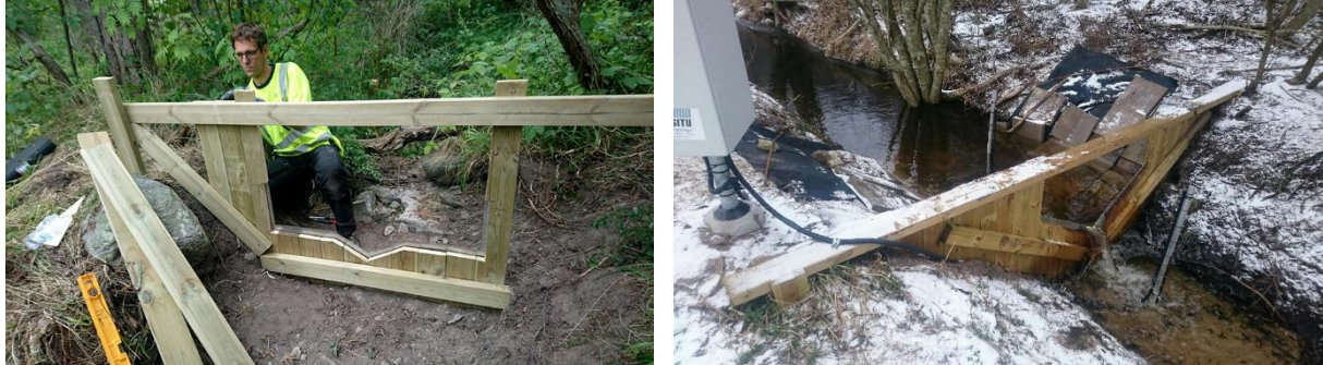
Figure 114. Installations of measurements stations for flow in ditches.
