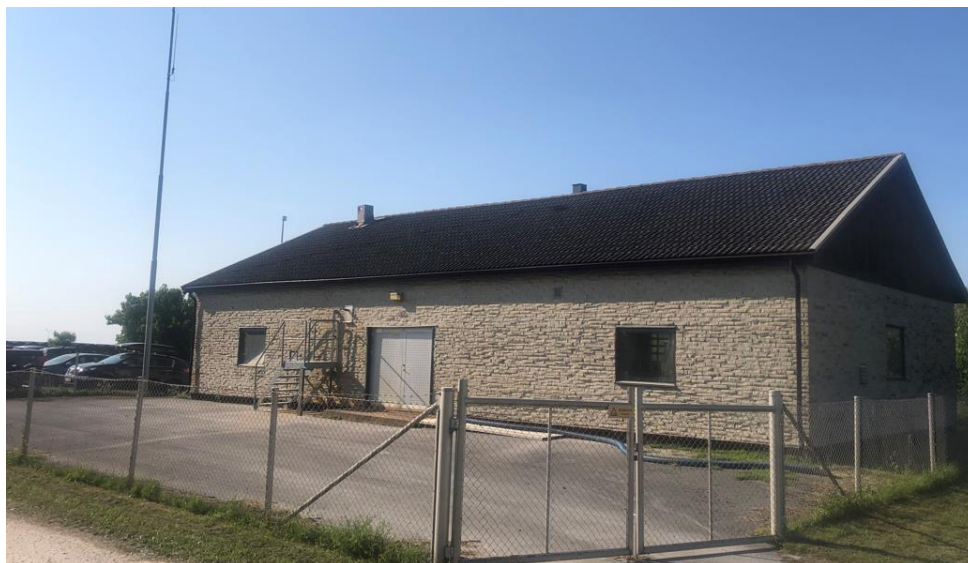
Figure 56. The former WWTP Burgsvik, now serving as the pilot center in the case study.
