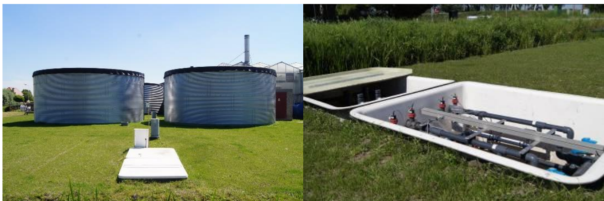
Figure 2. ASR system at Prominent in the Westland area. The aboveground water basins in combination with the ASR unit.
